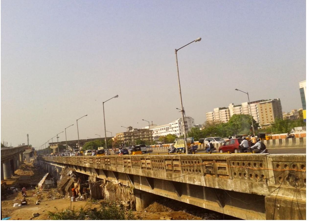
Maraimalai Adigal Bridge (Photo by R Muthusamy)
